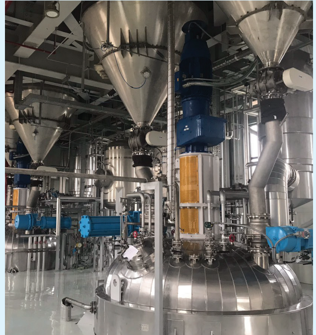
Install Equipment of Phenikaa Project
