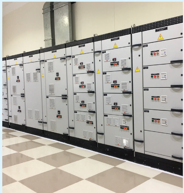
Install Control Panel of Phenikaa Project
