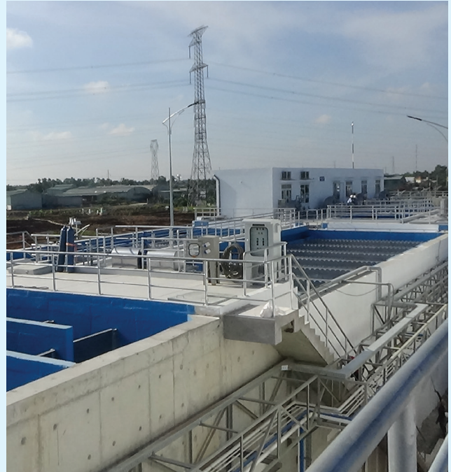
Install Equipment of Nhi Thanh Water treatment Plant Project
