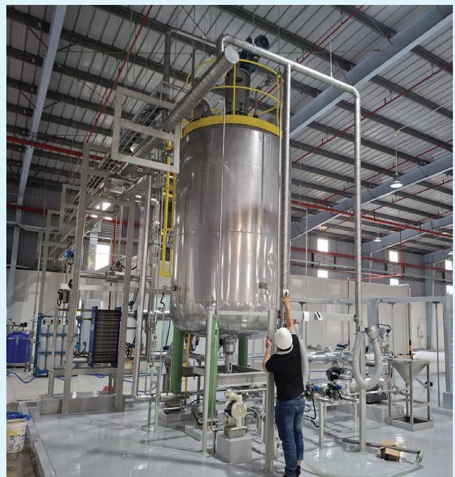
Install Piping of Blending Production Plant (PEARL)
