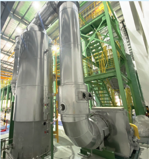
Install Equipment of Soda-VREC
