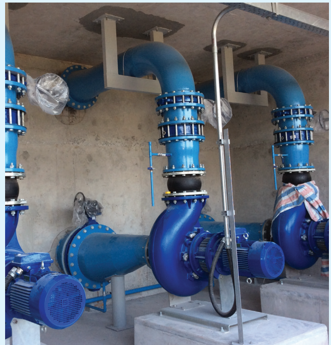
Install Piping of Yen Binh Water Treatment Plant Project
