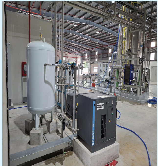
Install Equipment of Blending Production Plant (PEARL)
