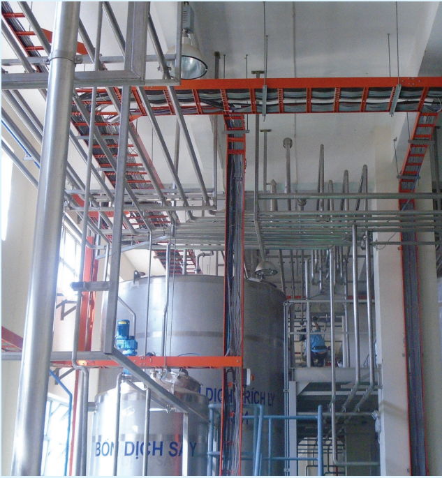
Install Piping of Long Thanh Vinacafé Project
