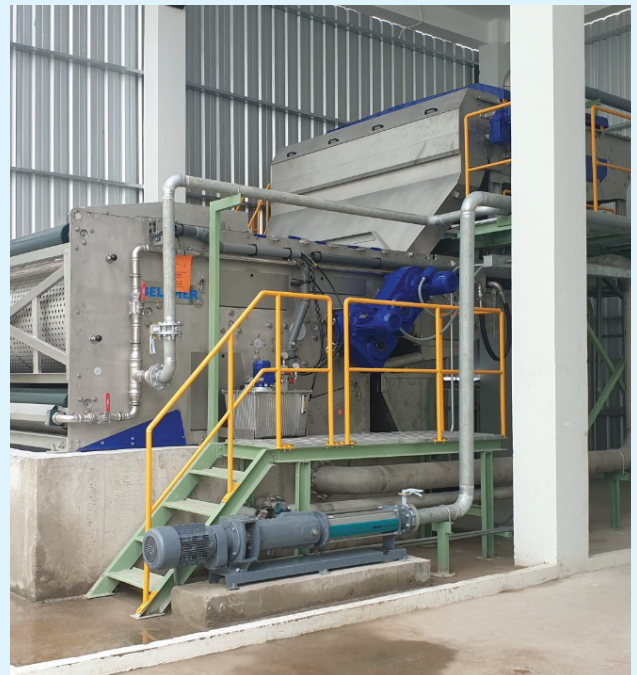
Install Equipment of Marubeni Kraft Paper Project
