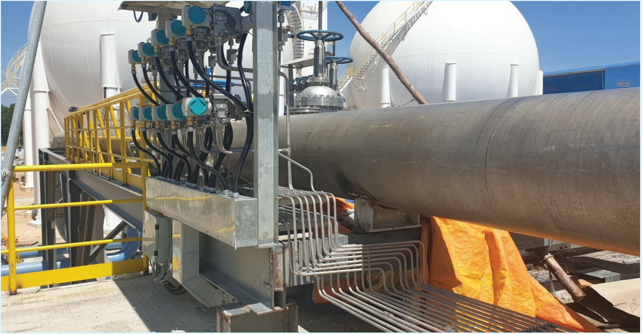
Install Instrument of Hoa Phat Quang Ngai Project
