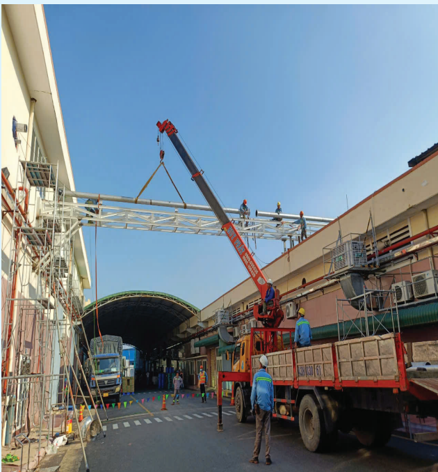
Install Piperack of Acecook Da Nang Project
