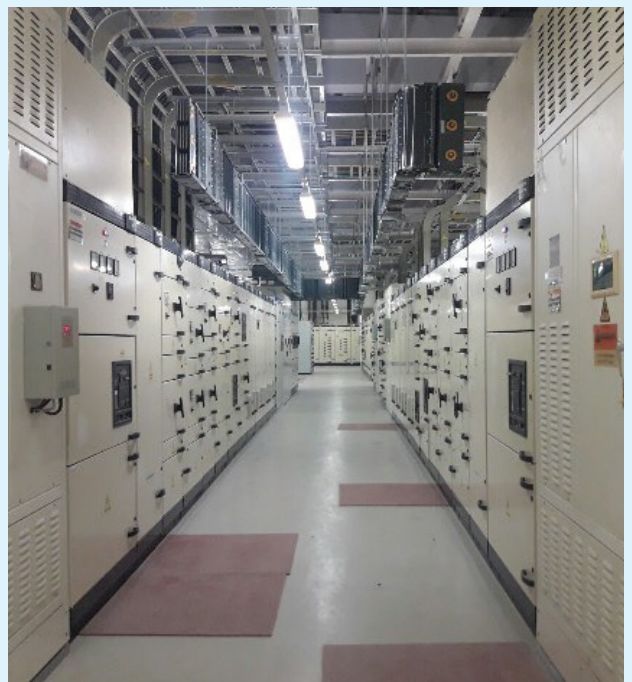
Install Control Panel and Busway of Intel Project
