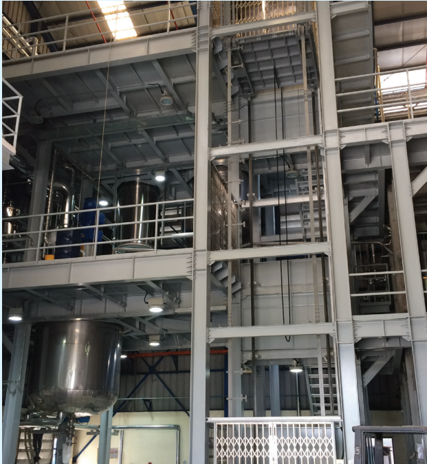
Install Equipment of Konishi Lemindo Project
