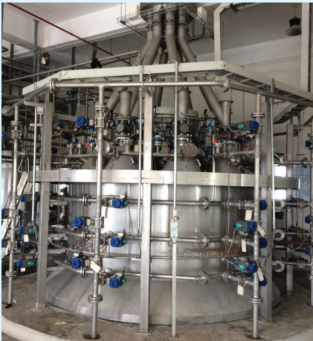
Install Equipment of Intimex Coffee Project
