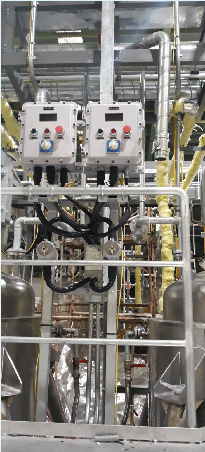
Install Electric Systems of Toyo Ink Project
