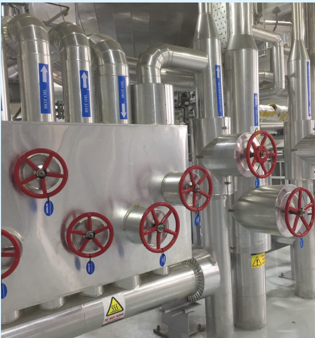
Install Piping of Intimex Coffee Project
