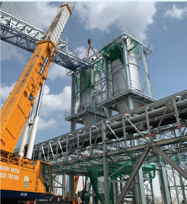
Install Equipment of Iguacu Coffee Project
