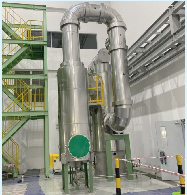
Install Equipment of Soda-VREC
