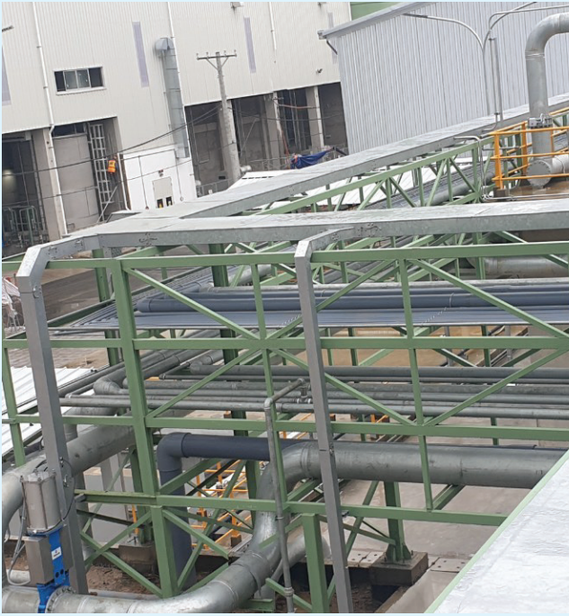
Install Piping of Marubeni Kraft Paper Project
