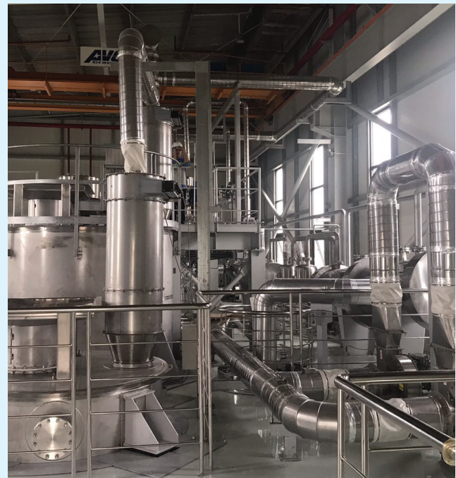
Install Piping of Phenikaa Project
