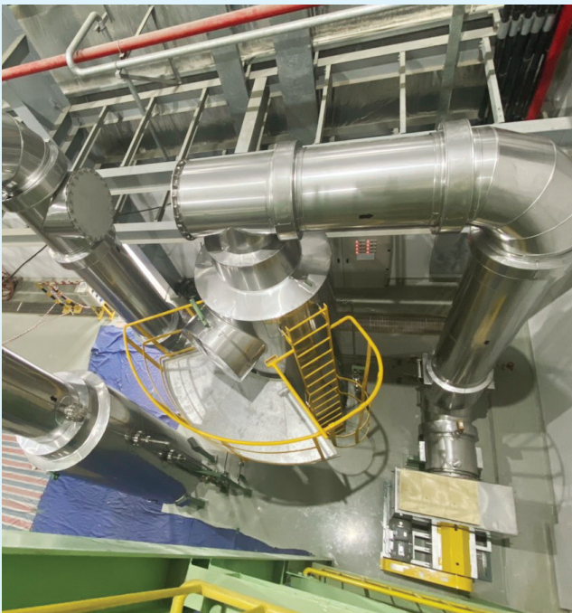
Install Piping of Soda-VREC
