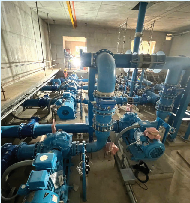
Install Piping of Water Supply System In Ta Khmau - Cambodia Project
