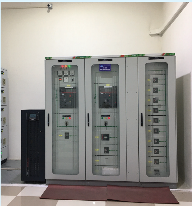
Install Control Panel of Phenikaa Project
