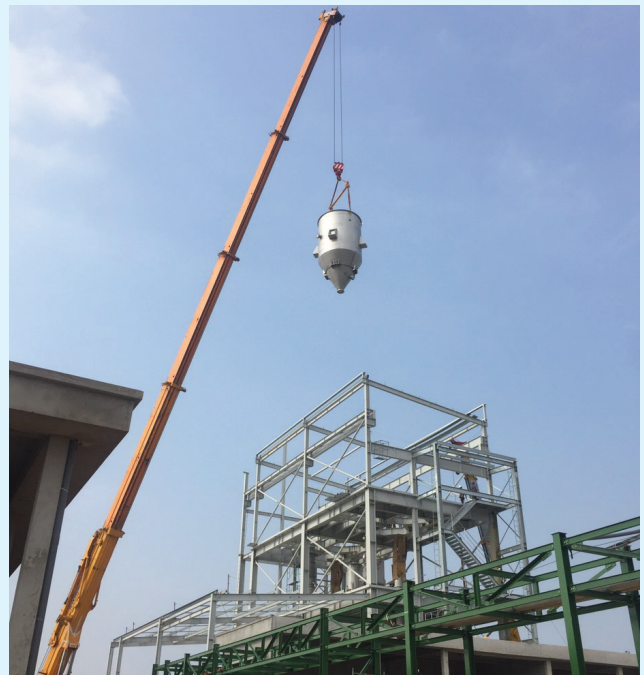
Install Equipment of Phenikaa Project
