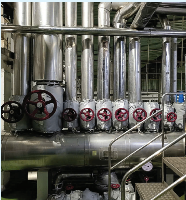
Install Piping of Acecook Da Nang Project
