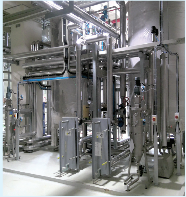
Install Piping of Iguacu Coffee Project
