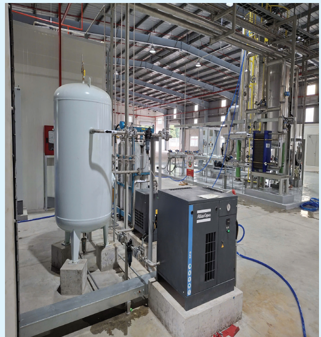
Install Equipment of Blending Production Plant (PEARL)
