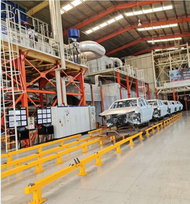
Install Equipment of Mercedes - Benz Vietnam Project
