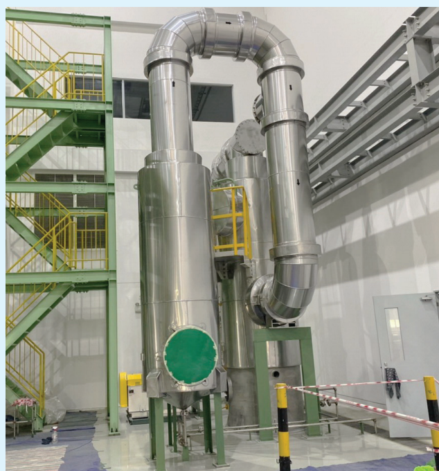
Install Equipment of Soda-VREC
