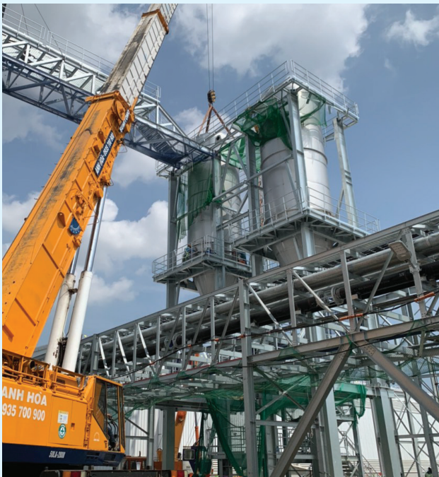
Install Equipment of Marubeni coffee Project
