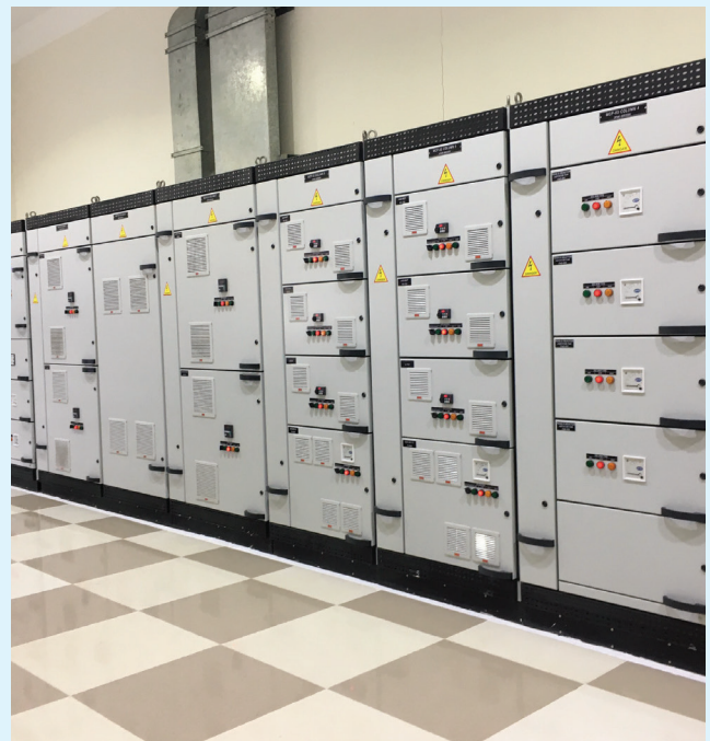
Install Control Panel of Phenikaa Project
