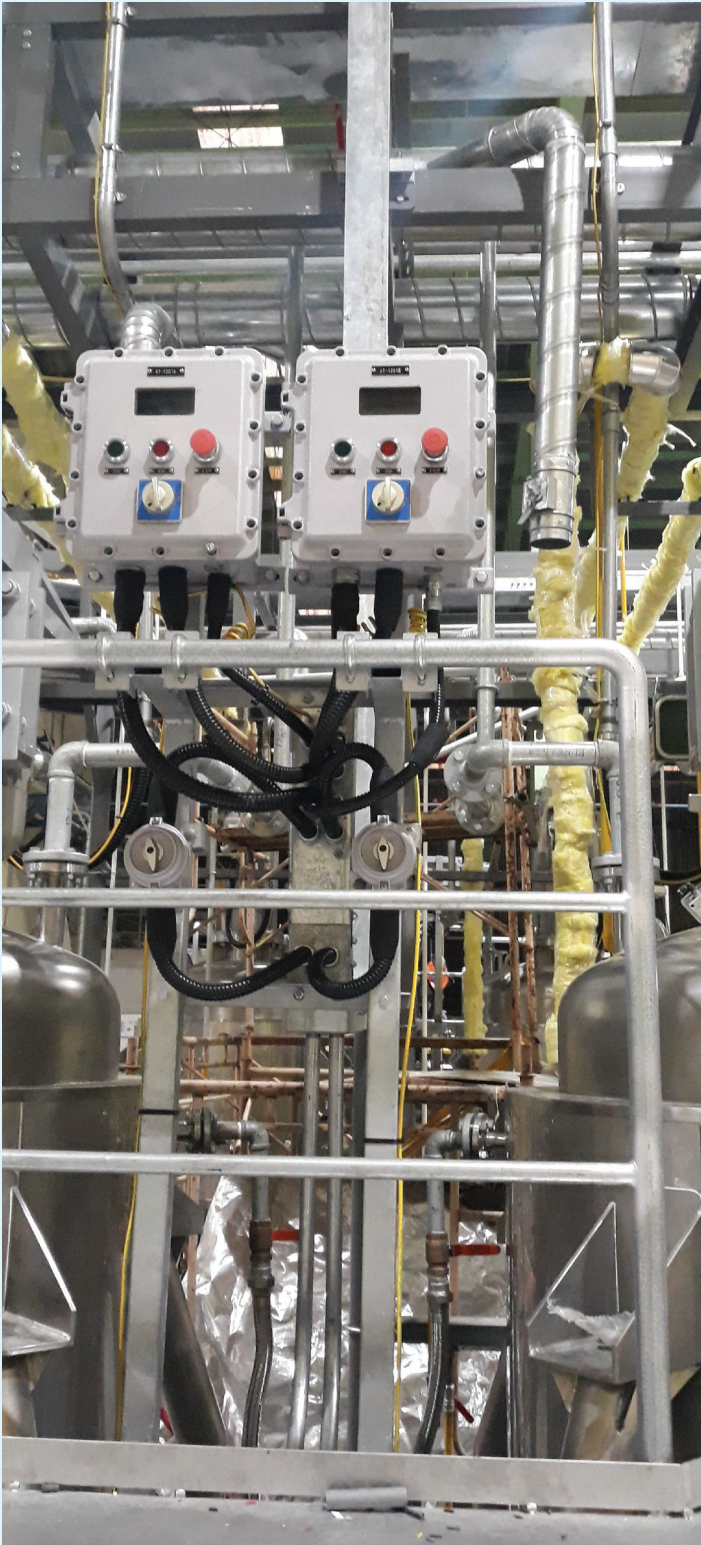
Install Electric Systems of Toyo Ink Project
