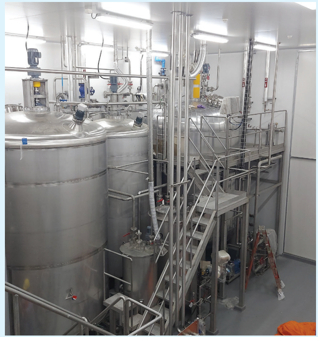
Install Piping of Semba Tohka Project
