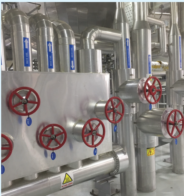
Install Piping of Intimex Coffee Project
