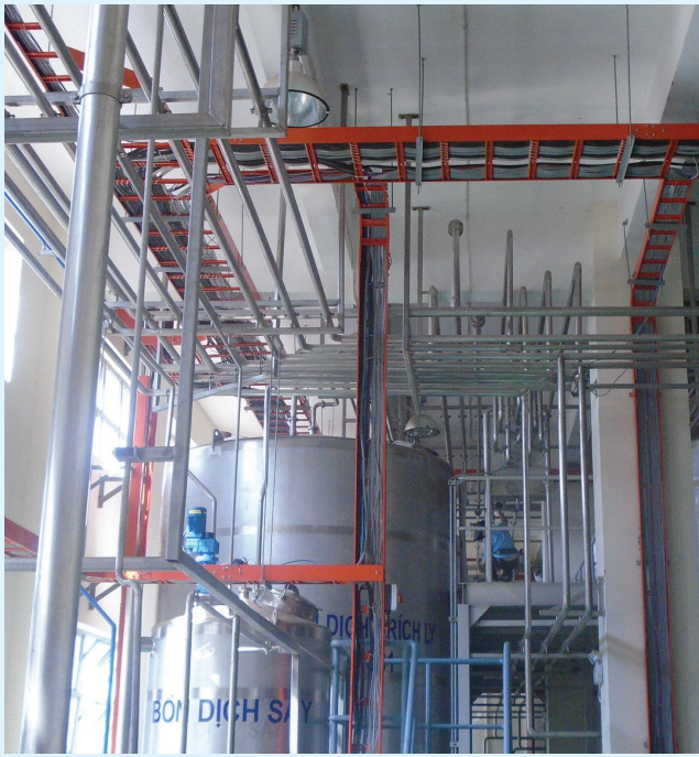
Install Piping of Long Thanh Vinacafé Project
