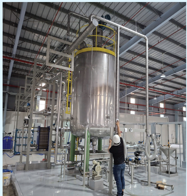
Install Piping of Blending Production Plant (PEARL)
