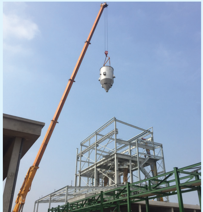
Install Equipment of Phenikaa Project
