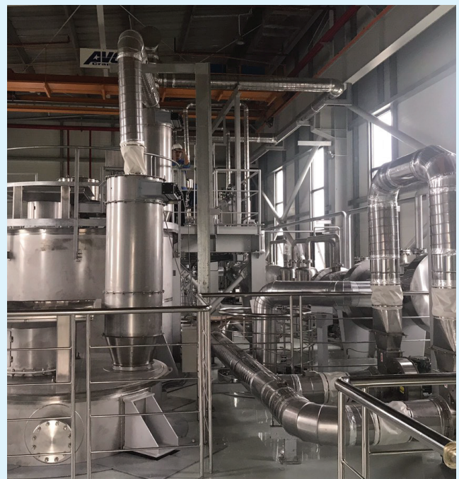
Install Piping of Phenikaa Project
