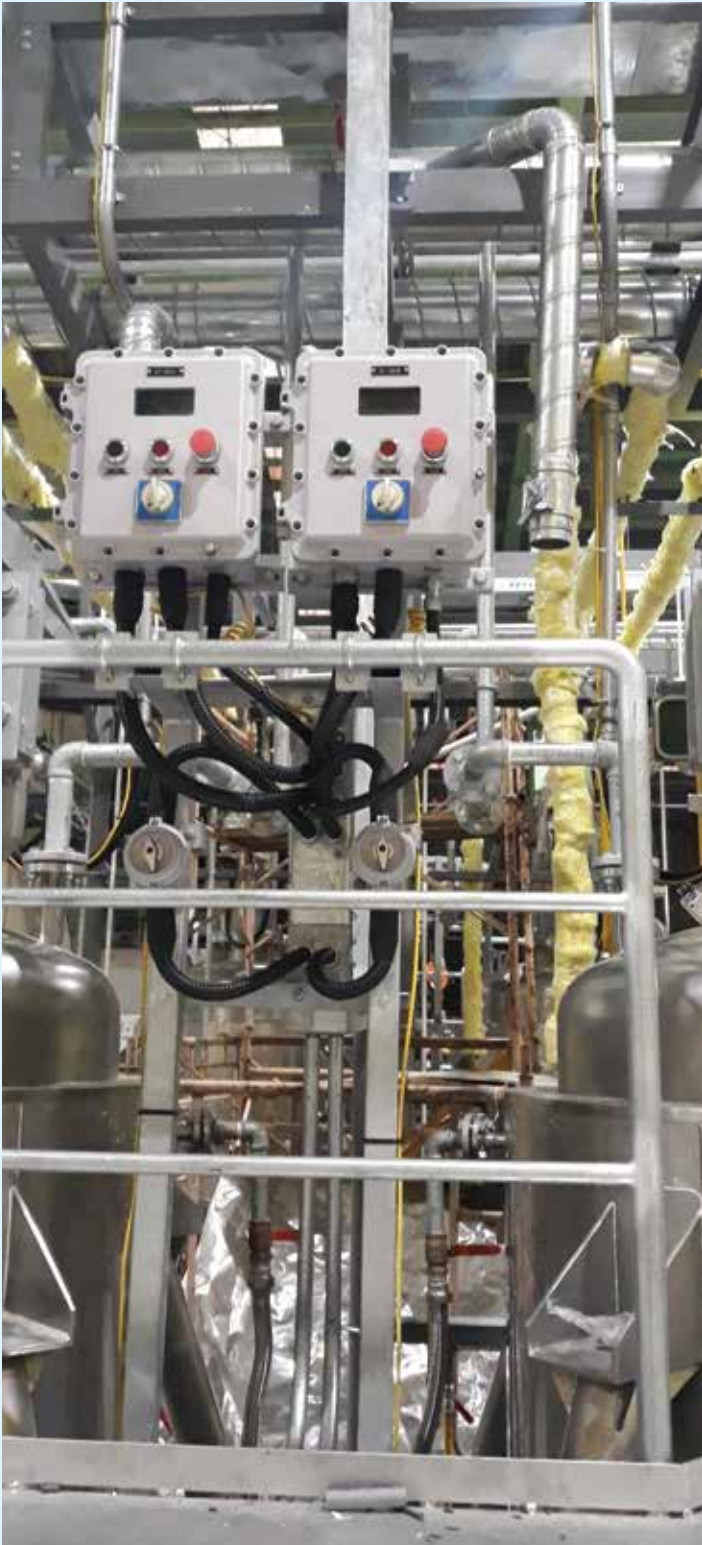
Install Electric Systems of Toyo Ink Project
