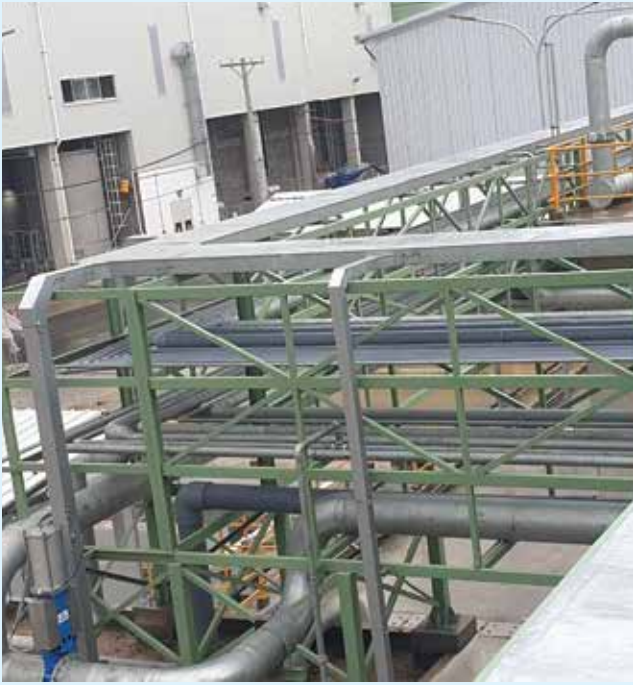
Install Piping of Marubeni Kraft Paper Project
