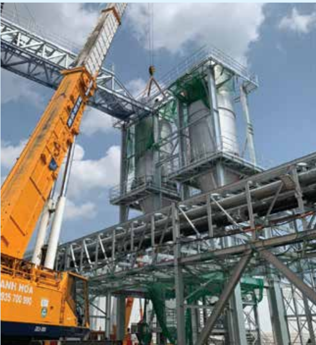
Install Equipment of Marubeni coffee Project
