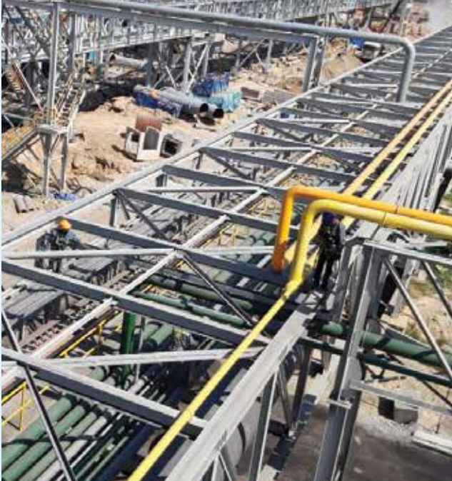
Pulling Cable and install instrument for Hoa Phat Project
