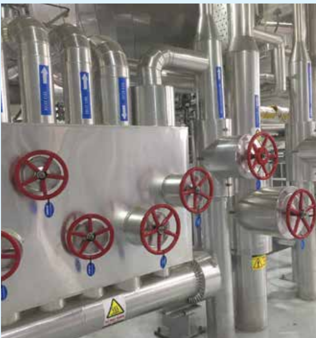
Install Piping of Intimex Coffee Project
