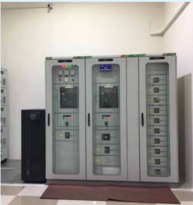
Install Control Panel of Phenikaa Project
