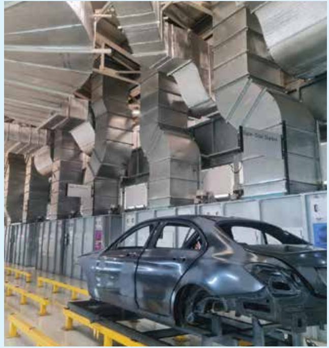
Install Duct Pipe of Mercedes - Benz Vietnam Project
