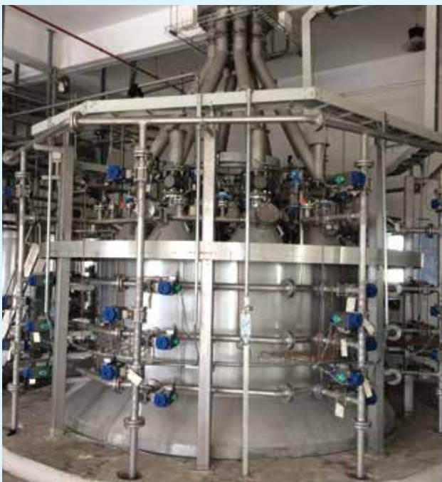
Install Equipment of Intimex Coffee Project
