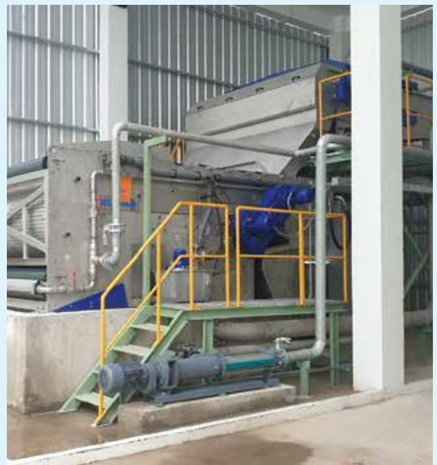
Install Equipment of Marubeni Kraft Paper Project
