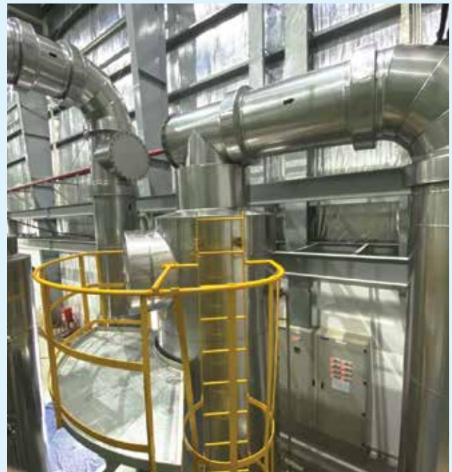
Install Piping of Soda-VREC
