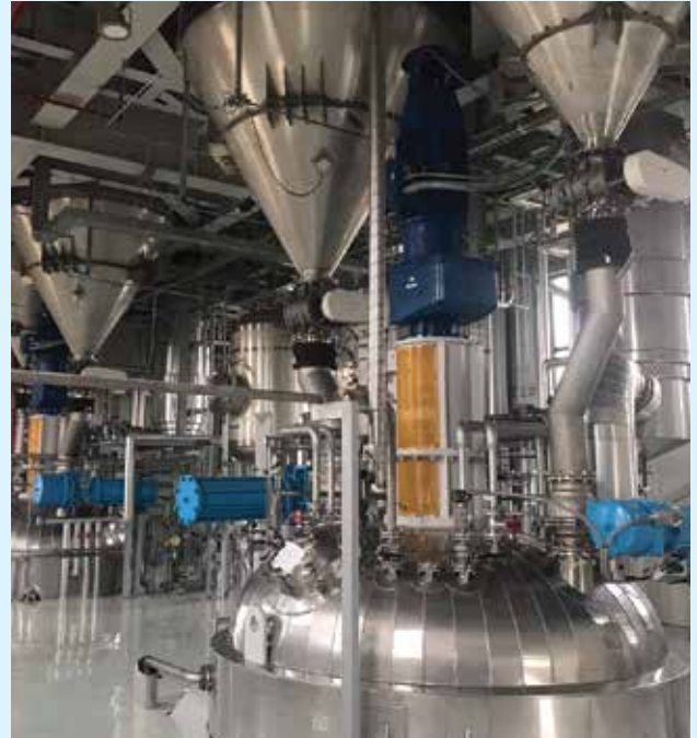
Install Equipment of Phenikaa Project
