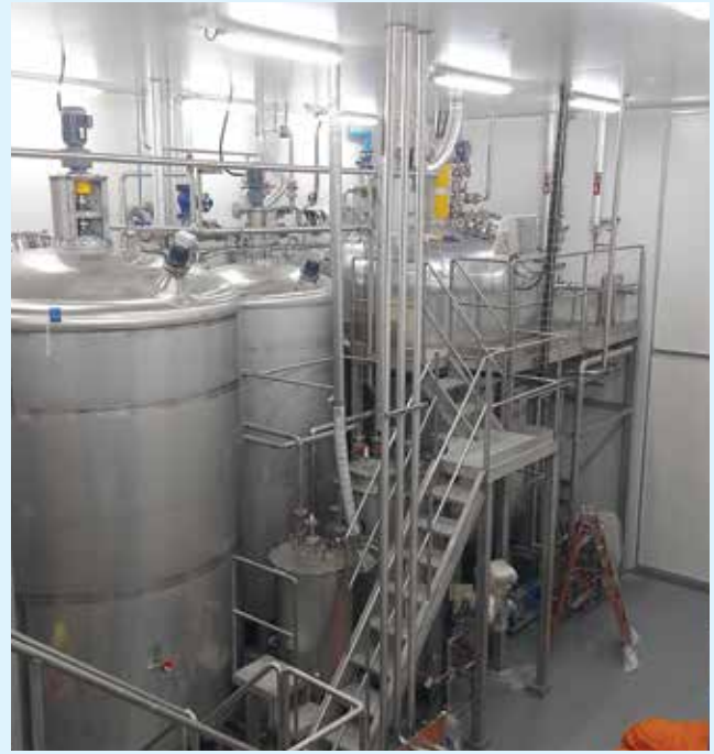
Install Piping of Semba Tohka Project
