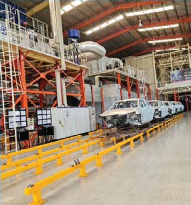
Install Equipment of Mercedes - Benz Vietnam Project
