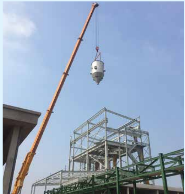
Install Equipment of Phenikaa Project
