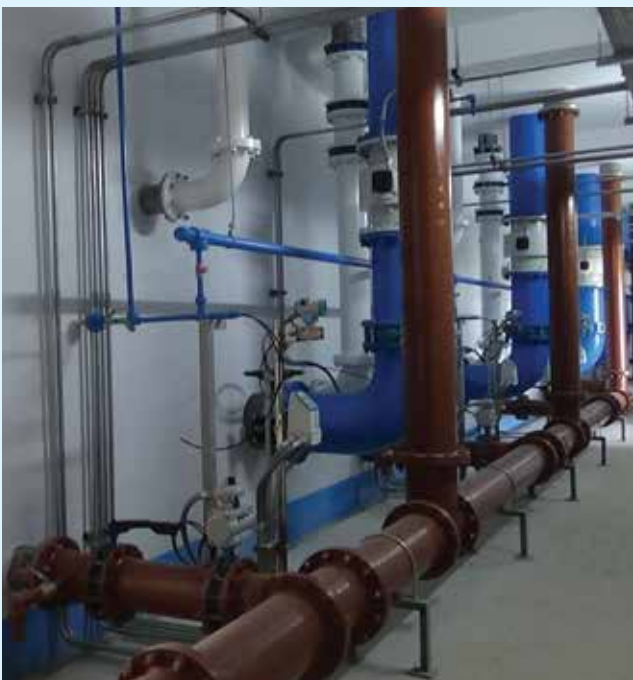
Install Piping of Nhi Thanh Water Treatment Plant Project
