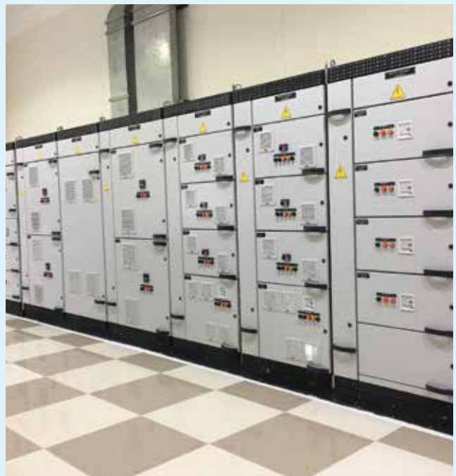
Install Control Panel of Phenikaa Project
