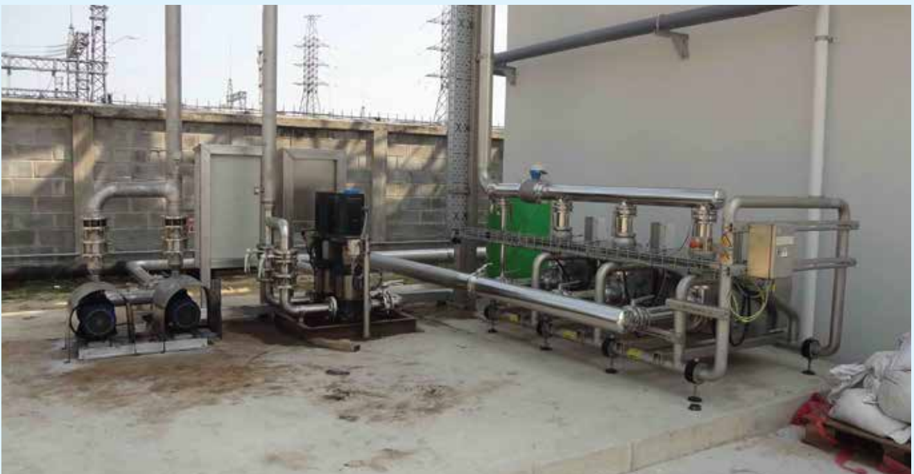
Install Electric System of Pepsico Quang Nam Project
