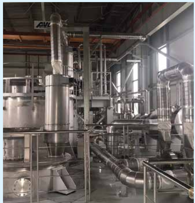
Install Piping of Phenikaa Project
