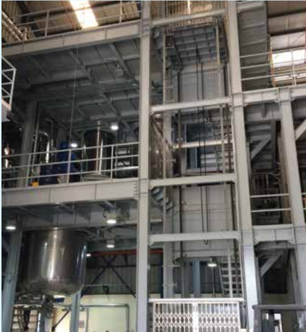
Install Equipment of Konishi Lemindo Project
