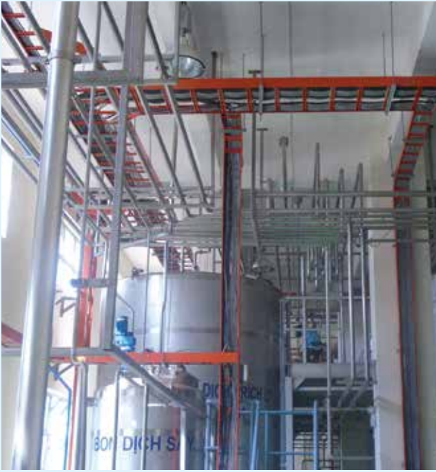
Install Piping of Bien Hoa Vinacafé Project
